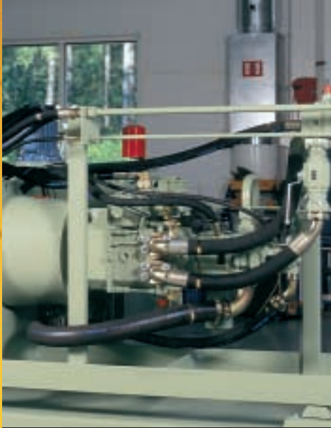
Less clogging and corrosion
